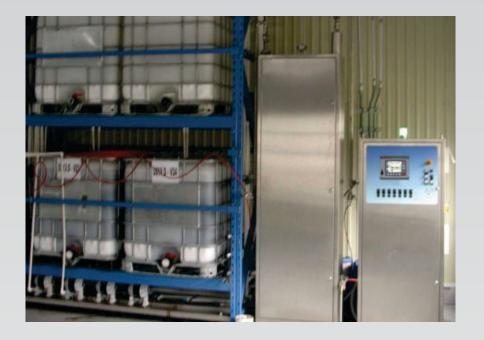
The whole system is made of stainless steel and allows to dose 98 % of the available chemicals used in the textile industry. All components (valves, flanges and piping) are specially designed for low contamination and fast wash out.
